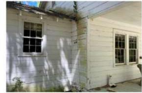
Figure 56. Lead Based Print on Extenor Siding
